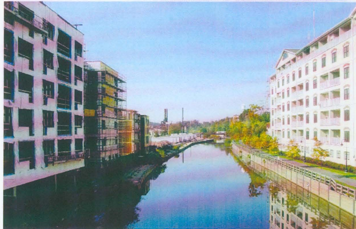
VIEW FROM LEVERINGTON AVE BRIDGE LOOKING AT ADJACENT PROPERTY
