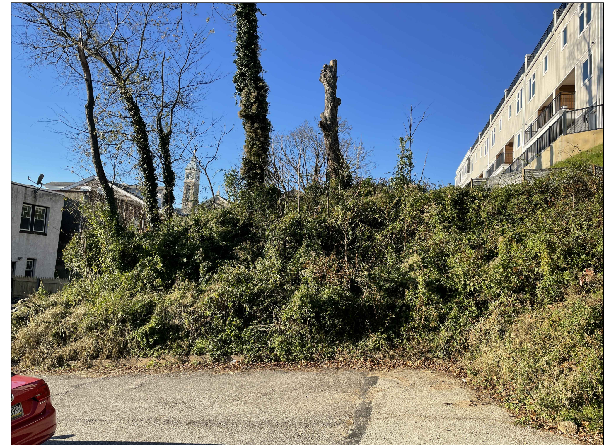
VIEW OF 251 RIPKA STREET
