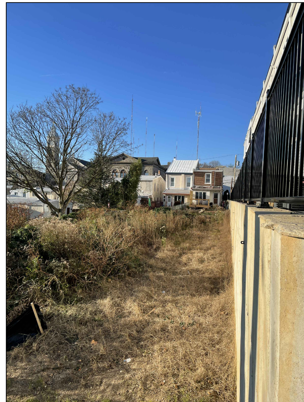
VIEW OF RETAINING WALL FOR NEIGHBORS TO THE WEST
