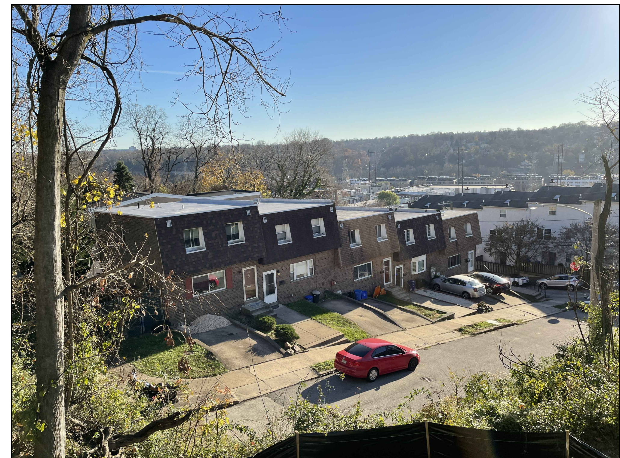
VIEW FROM 251 RIPKA LOOKING SOUTH
